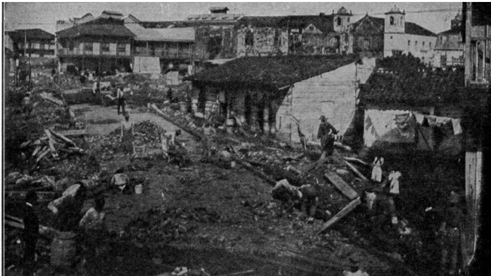
Figure 15. Street Paving Scene in Panama in Which an Old and Muddy Thoroughfare is Being Supplied with a Vitriified Brick Pavement Laid Upon Concrete , as illustrated in Theodore Roosevelt, Special Message of the President of the United States Concerning the December 17, 1906 (Washington, DC: United States Congress, 1906), n.p.
