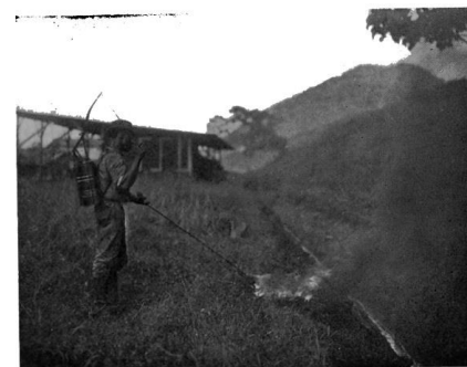
Burning Out Ditch With Oil Spray.
