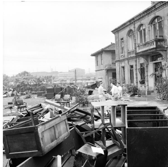
Fig. 5. Photograph showing the aftermath of the destroyed US Embassy in Taipei, 1957. Government Information Office, Executive Yuan, Taiwan
