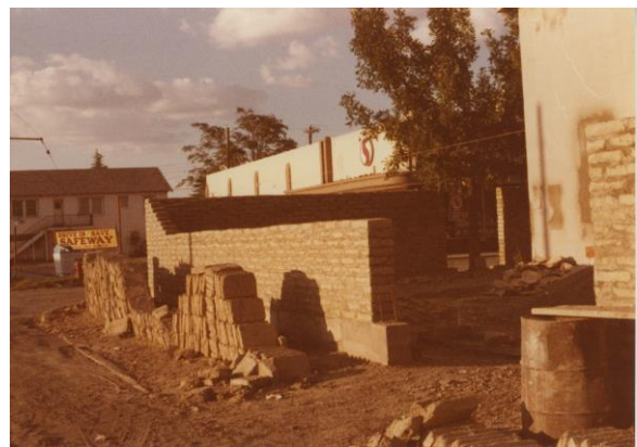
Fig. 21. Adobe/cement wall under construction for the Chinati Foundation's John Chamberlain building, 1979/80. Image courtesy of the Chinati Foundation Archives
